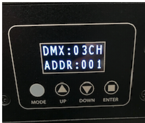
DMX CABLE CONNECTED
