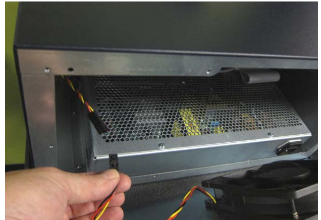
Disconnecting the fan cable
