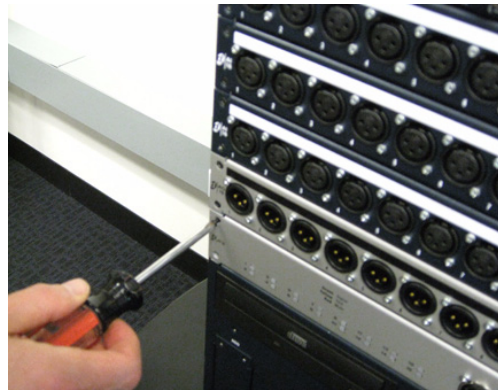
Securing an A-Net Card to Mix Rack's back panel
