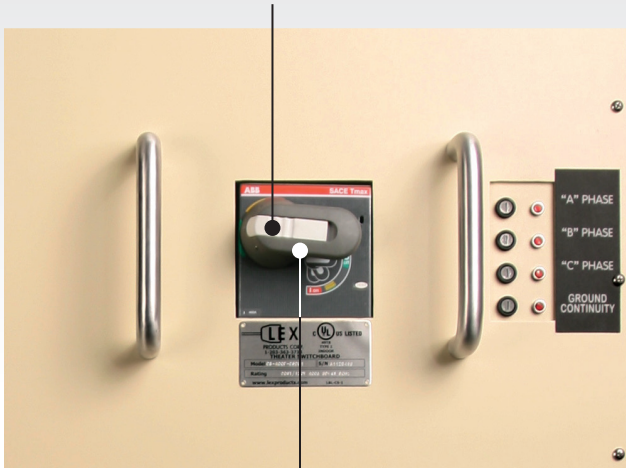
100% Rated electronic circuit breaker: 65,000 AIC Rating
