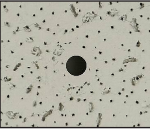
Fig A. Remove ceiling tile and drill 5/8" (16mm) hole in the desired location.
