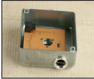
Fig B. Position the JBM3 plenum rated junction box 2 over the drilled hole.
