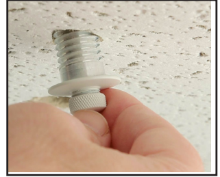
Fig C. Remove the nut from the threaded portion of the M3 cable 1 , feed cable through the tile hole and into the junction box.
