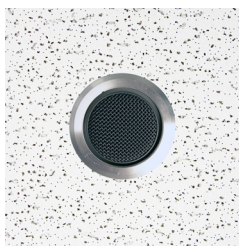
View looking up at ceiling with M3G6 microphone stored
